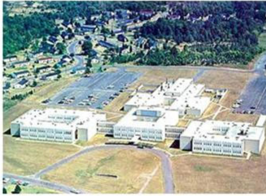
The SOE in 1964, the original complex was four interconnected buildings
